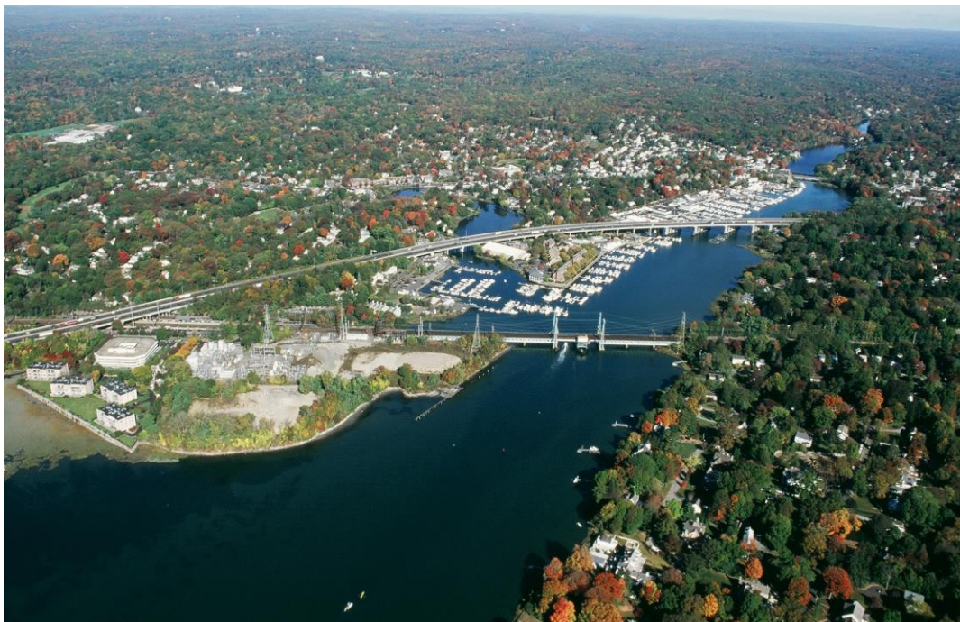
Photo 6-4: Cos Cob Harbor on the Mianus River; Cos Cob Park site prior to construction
