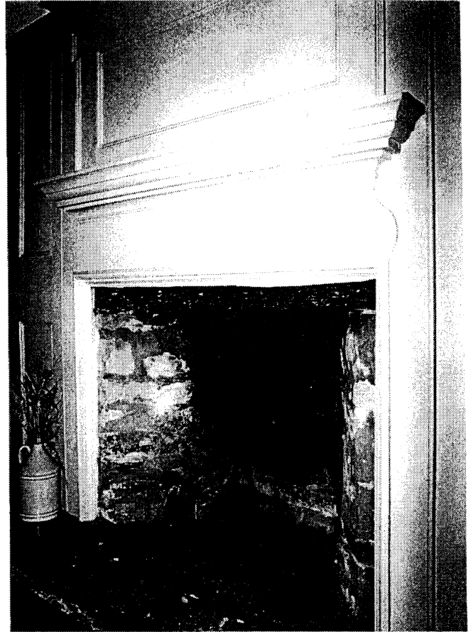
The paneling in the circa-1790 Titus Knapp house on Quintard Avenue has a characteristic design for its time, including the molded mantel shelf and a carved overmantel ornamented with corner "ears."
